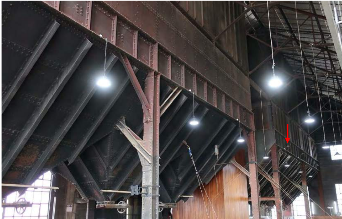
Boiler bay showing coal hoppers and original light fittings (indicated)
