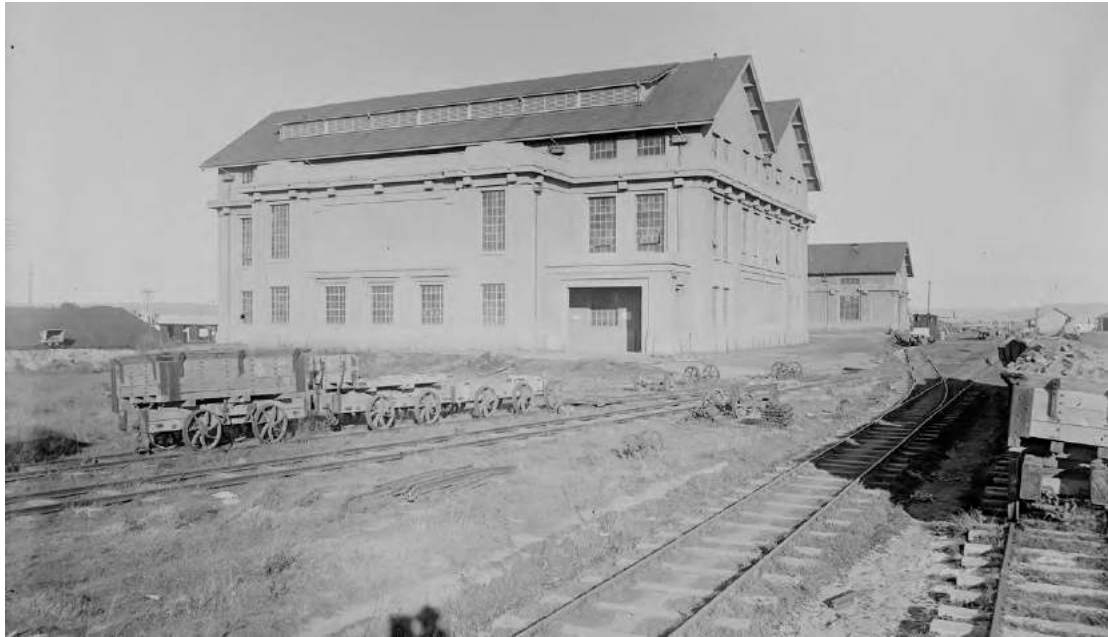
3 feet 6 inch Brickworks tracks and tipping wagons for disposal at the end of life of the Brickworks to Kingston railway. The central line terminated at the temporary engine shed evident behind the right wagon (1926) (Source: National Archives of Australia, A3560, 141)
