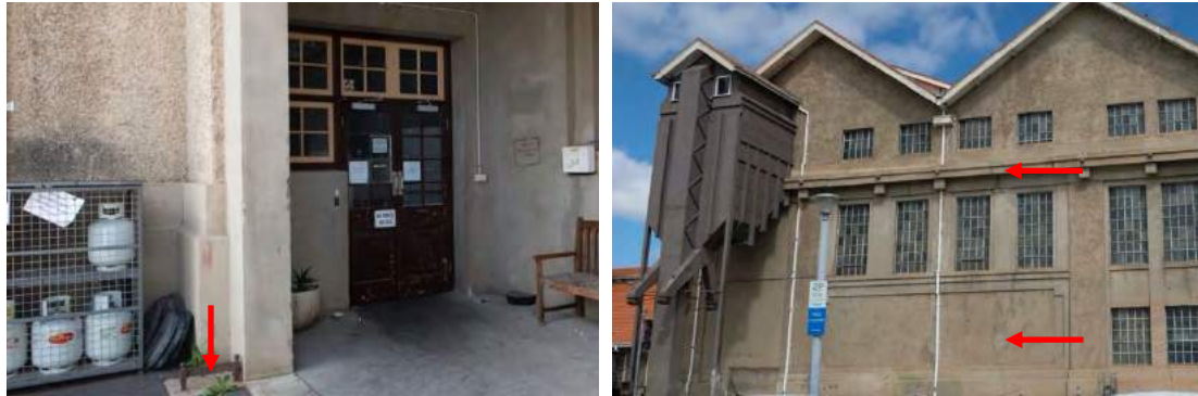
Left: Timber door to porch and boot scraper (red arrow). Right: Ash hopper and coal elevator to north-east end of boiler bay. The repair patches indicated (red arrows) is where the flue from the condenser pit penetrated the wall
