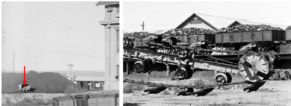
Left: Narrow gauge (2 feet) tipping skip at coal heap (1926)
