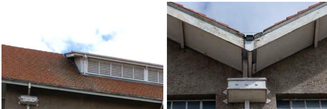
Left: Shed dormer/ventilator. Right: Rainwater head and decorative timber moulding to bargeboard
