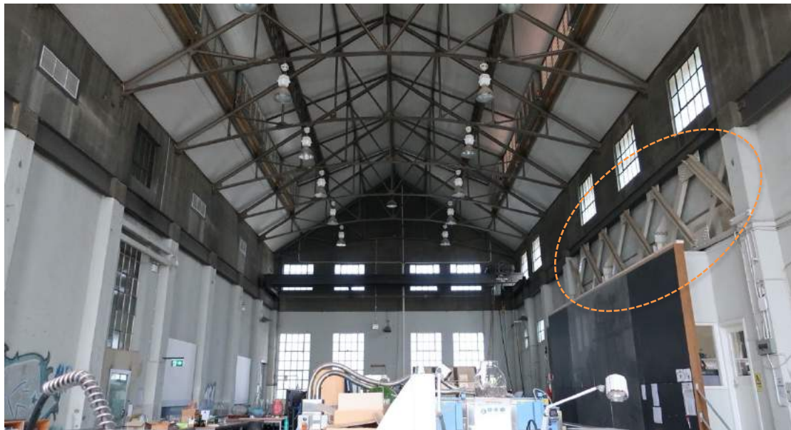
Engine bay looking south-west. The overhead crane is located adjacent to the far wall and the lattice girder above the opening to the former switchboard platform is indicated
