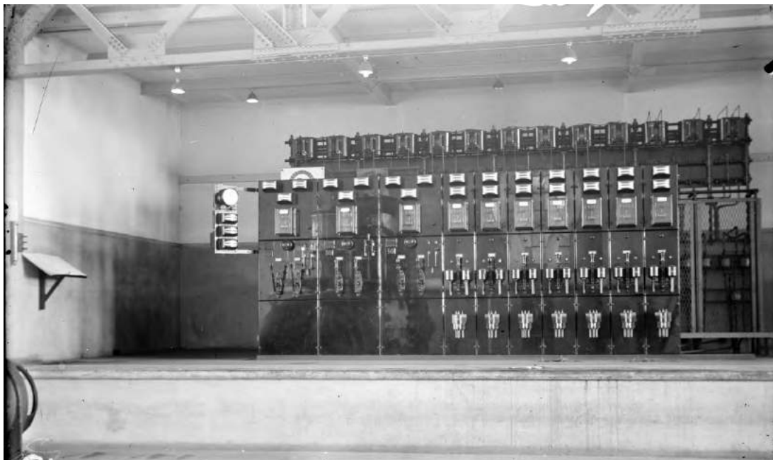
5.5kV switchboard on a raised platform in the engine bay (1926) (Source: National Archives of Australia A3560, 13)
