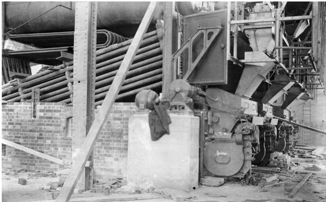
The fourth Babcock and Wilcox boiler under construction. Note the superheater and bank of water tubes below the steam and water drum. The motor drive for the chain grates is in the centre of the image (circa 1914) (Source: National Library of Australia, 143675733)
