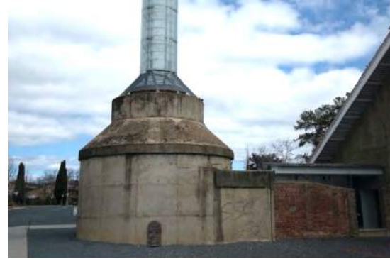
Left: Red brick interpretative device for original chimney. Right: Chimney base with red brick flue
