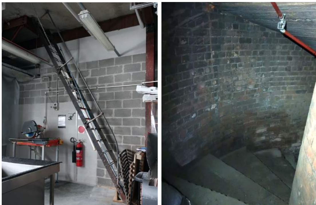
Left: steel ladder above location of condensing pits. Right: brick lined flue
