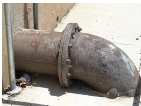
Left: Suction pipe penetrating the north-east wall of the Powerhouse at ground level Right: Design of circulating water outlet syphon (Source: Keith Baker and National Archives of Australia, A2445, M122)
