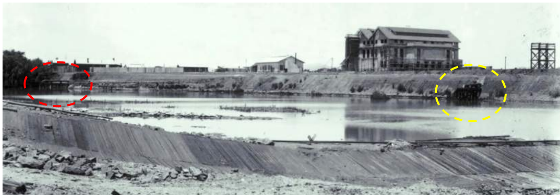
View of Powerhouse under construction showing the inlet pipe in red and the outlet pipe in yellow (circa 1914) (Source: National Library of Australia, 143676091)
