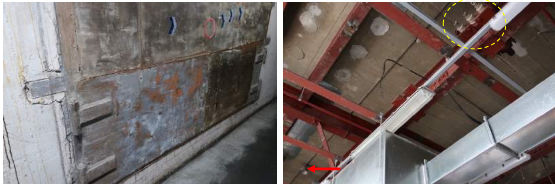
Left: steel doors to ash chute. Right: original light fitting (arrow) and cable terminating box (circle) to current mould making room
