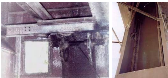
Left: Conveyor intermediate sprockets at north-east end above ash hopper. Right: Guide rails inside vertical conveyor duct (Source: Keith Baker)
