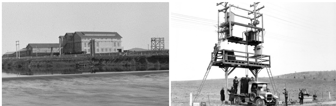
Left: Powerhouse with timber tower on right and 5.5kV Duntroon line on left (circa 1921-29)
