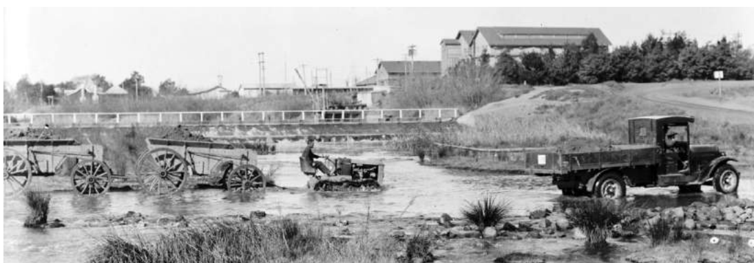
A more formally constructed weir with a handrail. The weir may have been higher than the previous and probably created a deeper pool upstream. A pump house also seems to have been constructed by this time (1928) (Source: National Archives of Australia, A3560, 4224)
