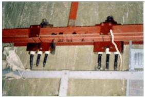
Cable terminations in cable chamber below high voltage switchroom
