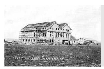
Figure 34. The Power House under construction in 1913, with Owen's galvanised iron 'temporary' Electrical Store and Machine Shop at right Source: CRS M77, image no. 31, National Archives of Australia
