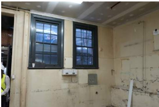
Left: south corner of former recreation room. Right: west corner of former recreation room showing damage to the hard plaster
