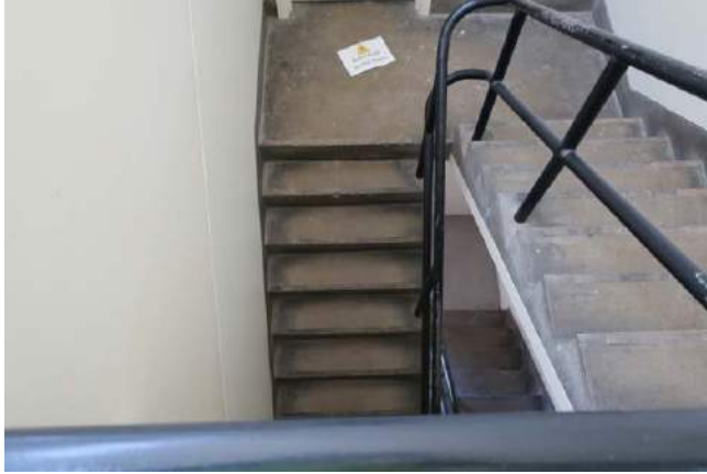
Concrete stair with pipe handrail
