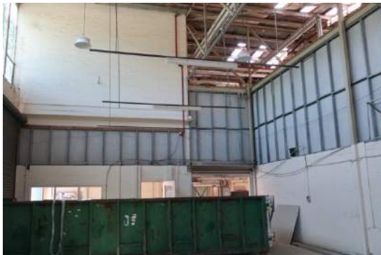
Left: modern partition above original brick walls. Right: green glazing to upper part of north-west gable end
