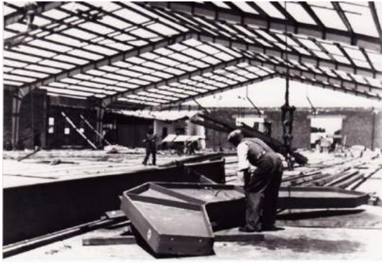
Left: portal frames being erected over the original open garage (circa 1941). Right: 1940s roof to original open garage (circa early 1940s)
