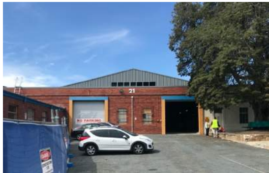
Left: north-west elevation of 1927 depot building with 1940 roof clad in modern corrugated sheeting. Right: west end of south-west elevation, 1927 depot with original steel framed windows and overpainted brickwork
