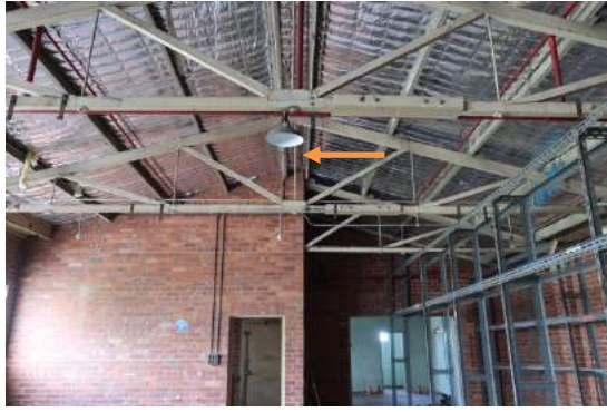
Left: Upper floor of 1951 workshop with original hoist (indicated) and timber doors.
