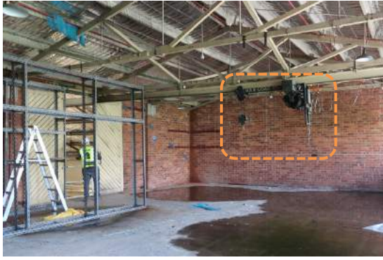
Left: Upper floor of 1951 workshop with original hoist (indicated) and timber doors.
