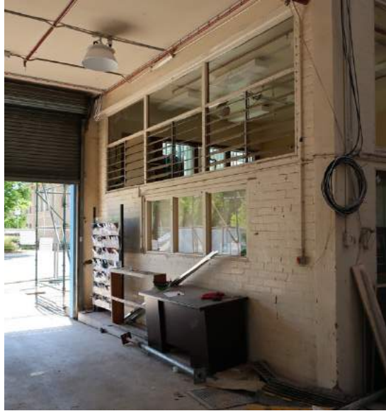
Left: south-east side of traffic office. Right: south-west side of traffic office with early glass louvers to the upper part
