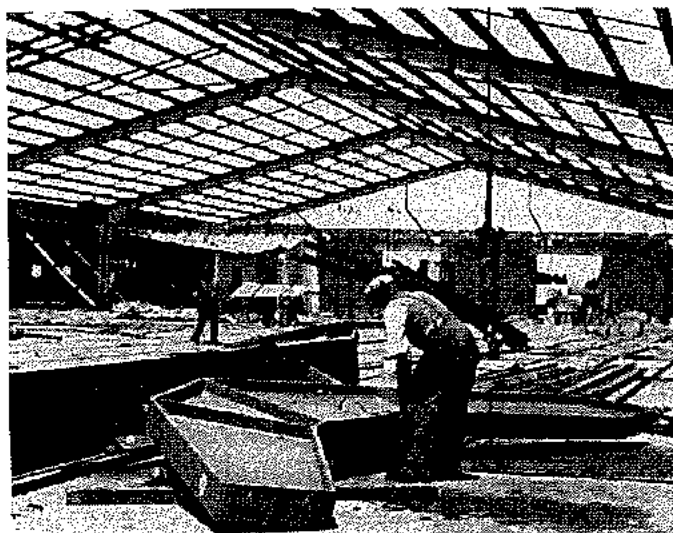
Plate 10: Inside the Depot looking southeast, with the fully welded rigid portal frame over the existing 'Garage' under construction, 1941. Source: Val Emerton. Jack Benson photograph.
