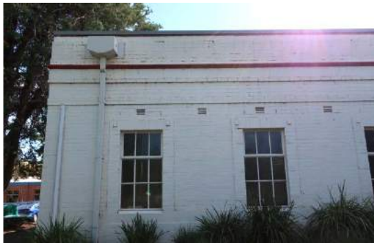
Left: north-west elevation of 1927 depot building with 1940 roof clad in modern corrugated sheeting. Right: west end of south-west elevation, 1927 depot with original steel framed windows and overpainted brickwork
