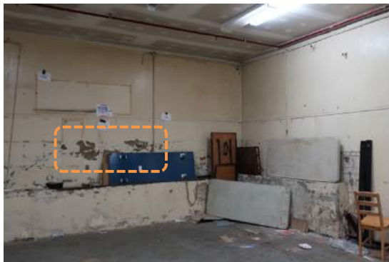
Left: south corner of former recreation room. Right: west corner of former recreation room showing damage to the hard plaster
