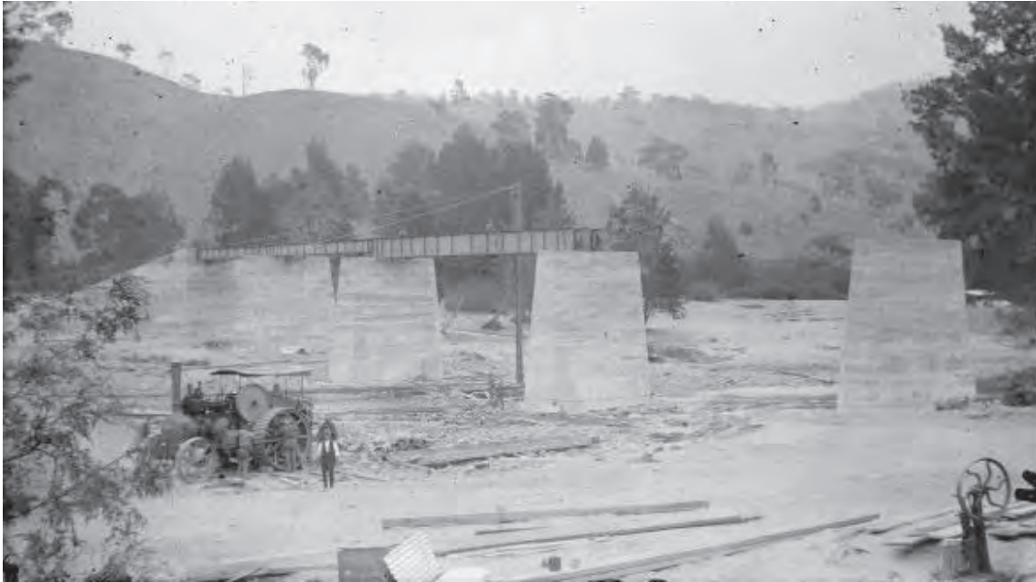
Figure 7 Construction of the bridge over the Murrumbidgee River, with a McLaren traction engine in the foreground c.1913 Source: National Library of Australia
