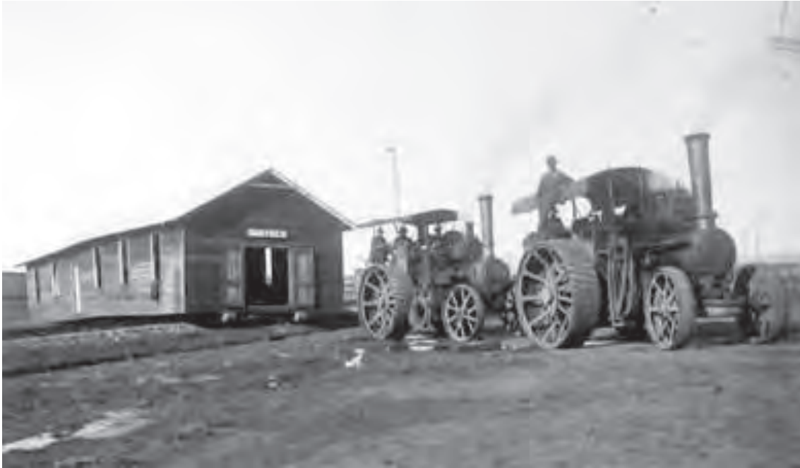
Figure 9 McLaren (left) & Fowler compound traction engines moving a timber canteen building from the Molonglo camp, Canberra Source: National Archives of Australia (Mildenhall Collection)
