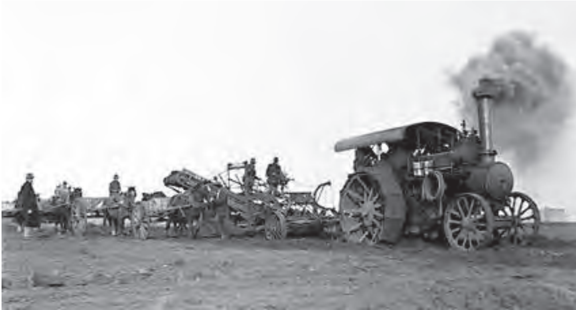
Figure 13 Another view of one of the two Fowler road locomotives at the South Ainslie business sites (c. Jan-June 1926): due to the soft ground the rear wheels are fitted with spuds (cleats) to improve traction Source: National Archives of Australia (Mildenhall Collection)
