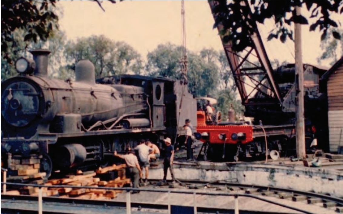
Figure 21 Fowler engine no 16161 pulling NSW railway locomotive no.5476 out of the locomotive turntable pit, Cowra, in 1966: the Fowler engine can be seen in the background Source: Bruce Macdonald collection
