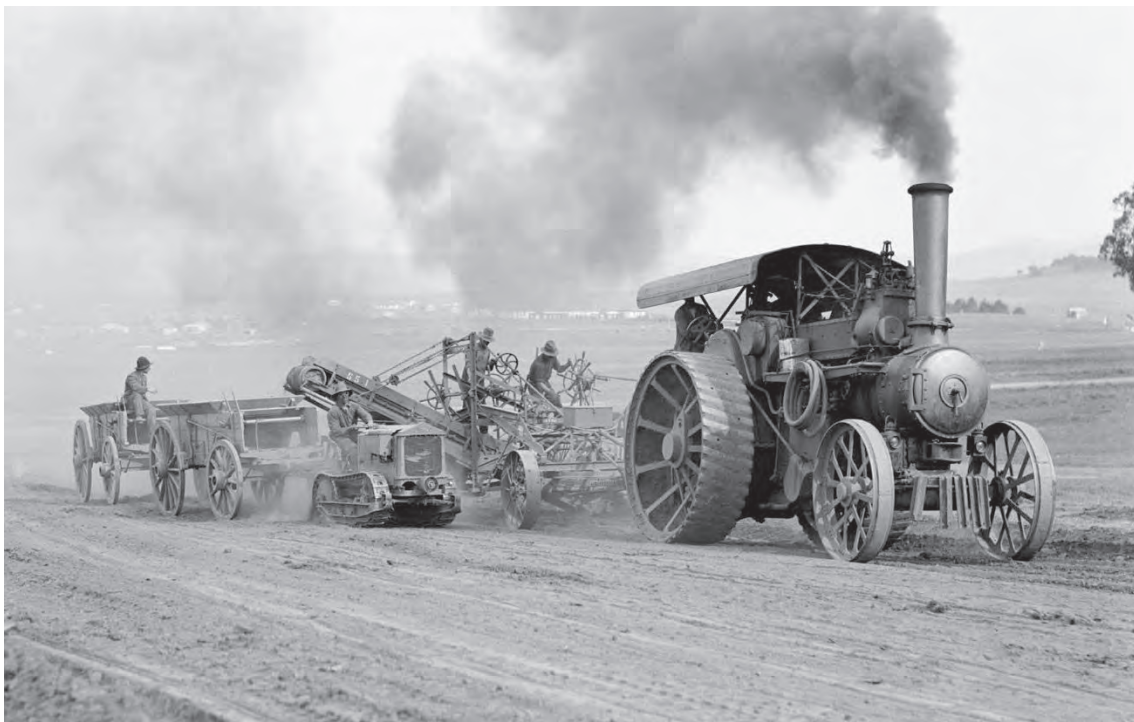
Figure 14 One of the Fowler road locomotives towing the New Era elevating grader while forming a road way Source: National Archives of Australia (Mildenhall Collection)
