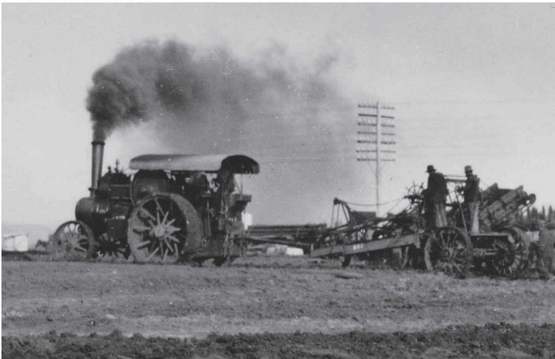
Figure 12 One of the Fowler road locomotives hauling a 'New Era' elevating grader at the South Ainslie business sites (c. Jan-June 1926) Source: National Archives of Australia (Mildenhall Collection)
