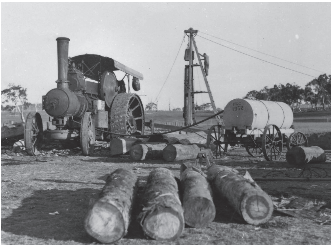
Figure 16 Fowler road locomotive no.16162 being used to drive piles for a bridge Source: National Archives of Australia (Mildenhall Collection)
