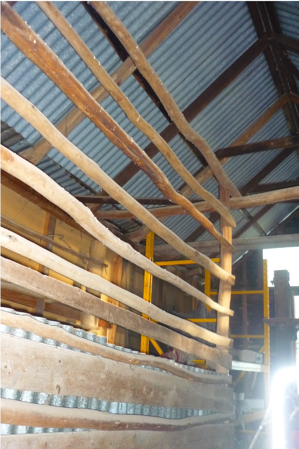
Image 23: Shows the bush poles of the tall wool sorting bins.
