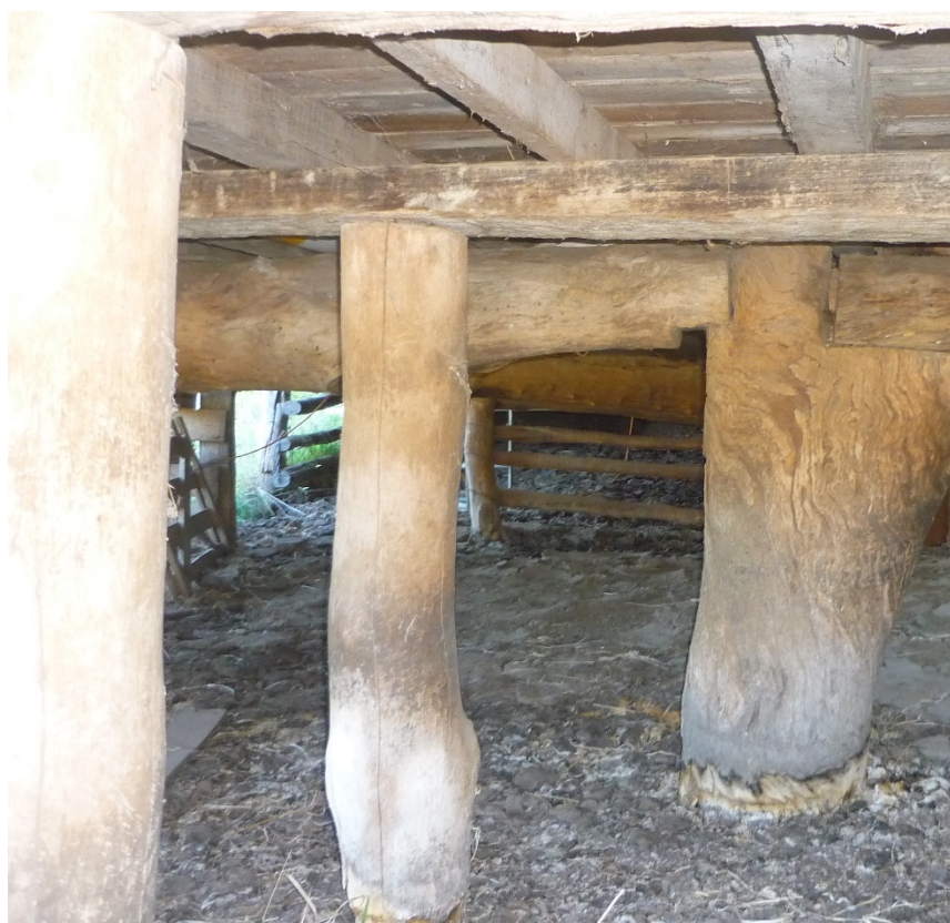
Images 25 – 27: Shows bush pole framing and top of tall wool sorting bins. Shows large framing timber and large timber and bush pole pens under the building.
