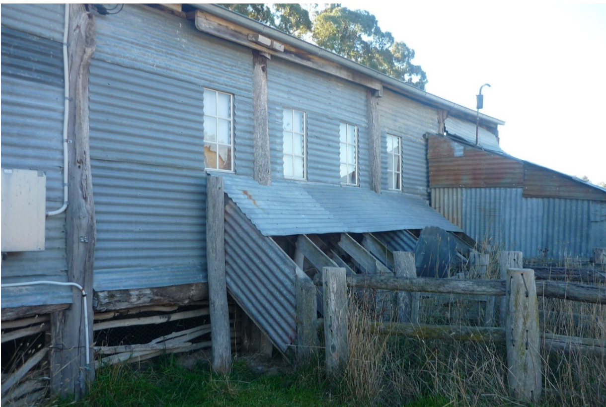
Image 28 and 29: The front of the woolshed. The bottom image shows the chutes from the shearing board to the tally pens. Can also see the car exhaust from the machinery shed roof.
