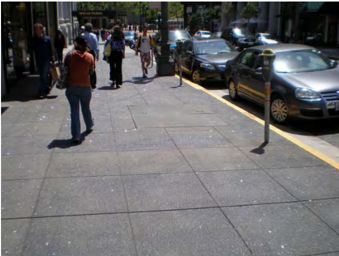
Dark grey insitu concrete paving with carborundum additive
