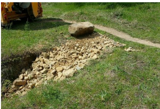
Stabilising a gully in Bullen Range Nature Reserve (PCS)
