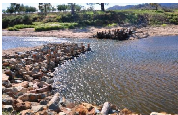
Engineered Log Jam downstream of Tharwa (Mark Jekabsons)
