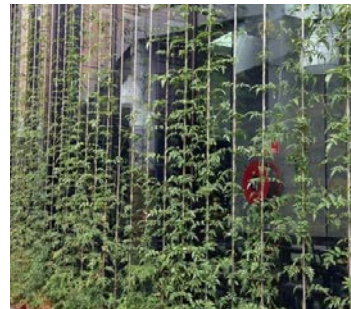
GALVANIZED WIRE ROPES FOR CLIMBERS
