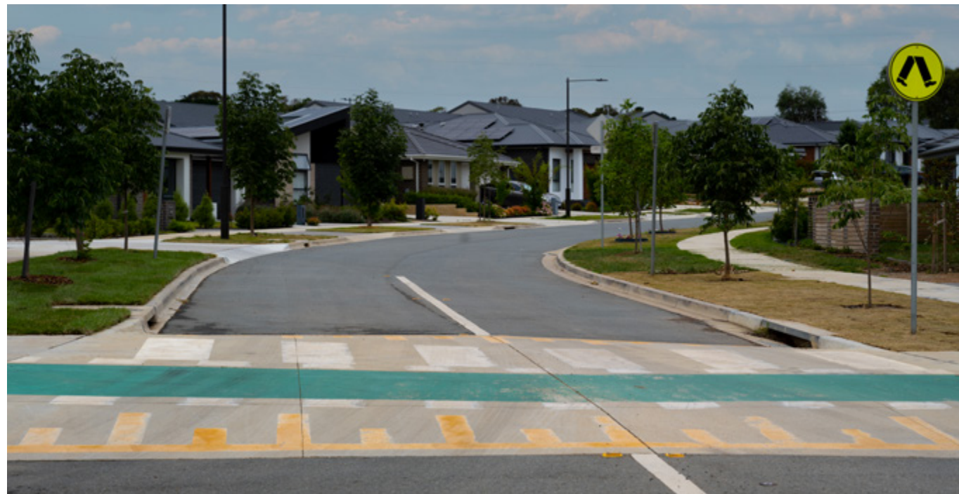
Figure 9 Raised priority/ zebra crossing with clear priority for walking and riding (note the green treatment indicates a cycleway adjacent to a footpath)
